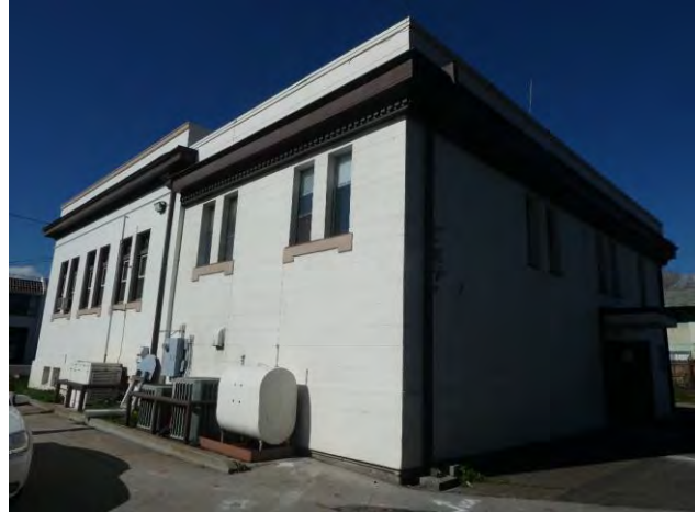
Figure 9: East elevation, view facing southwest. GPA 2022.
