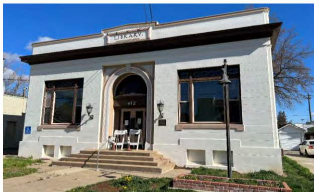
Figure 1: Primary elevation, view facing north. GPA 2022.
