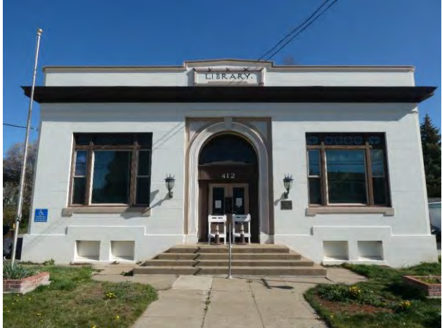
Figure 8: South elevation, view facing north. GPA 2022.
