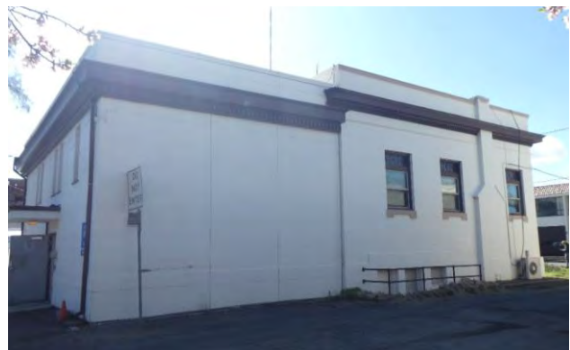
Figure 2: West elevation, view facing southeast. GPA 2022.
