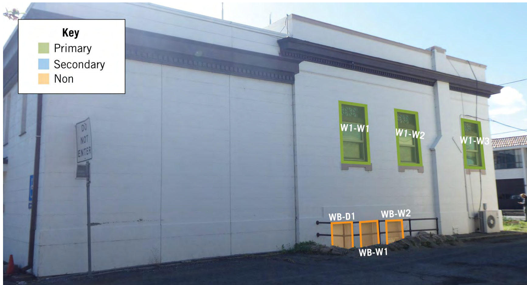
Figure 13: Windows and doors on west elevation. (GPA Consulting, March 2022).
