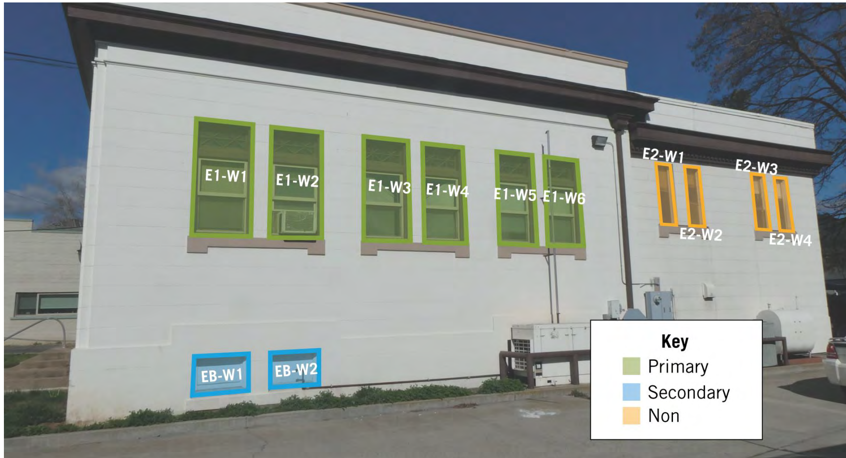
Figure 11: Windows and doors on east elevation. (GPA Consulting, March 2022).
