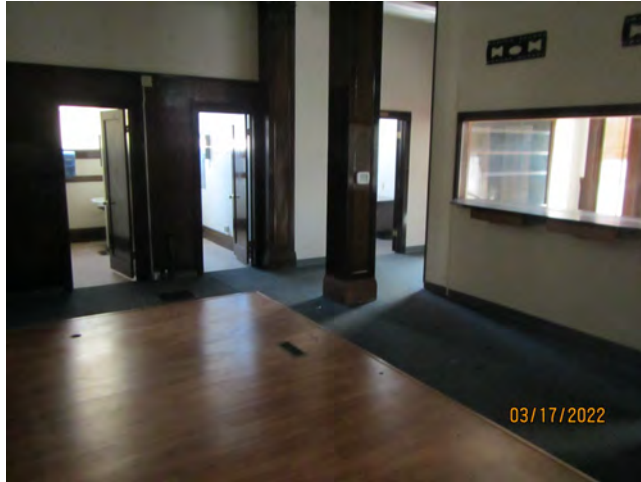
Photo 22 – Typical asbestos-containing gypsum board wall system, 1st floor, southern offices
