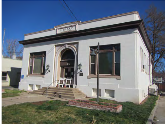
Photo 1 – Yreka Library building (southern exterior), 412 West Miner Street, Yreka, Siskiyou County, California
