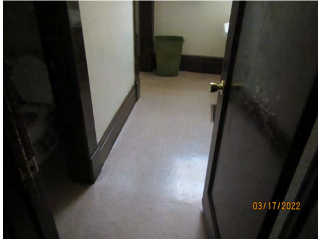
Photo 10 – Tan pebble-pattern resilient sheet flooring, 1 st floor, restrooms, southern offices
