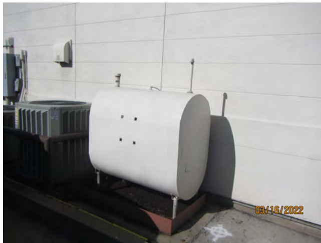
Photo 39 – Unused kerosene aboveground storage tank, eastern exterior
