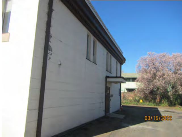
Photo 4 – Northern exterior of the site building
