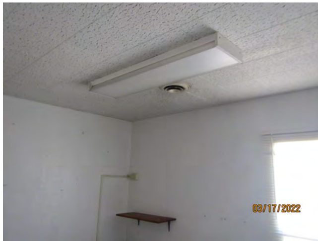
Photo 14 – Typical 12”x12” acoustical ceiling tiles, 2 nd floor, northern offices
