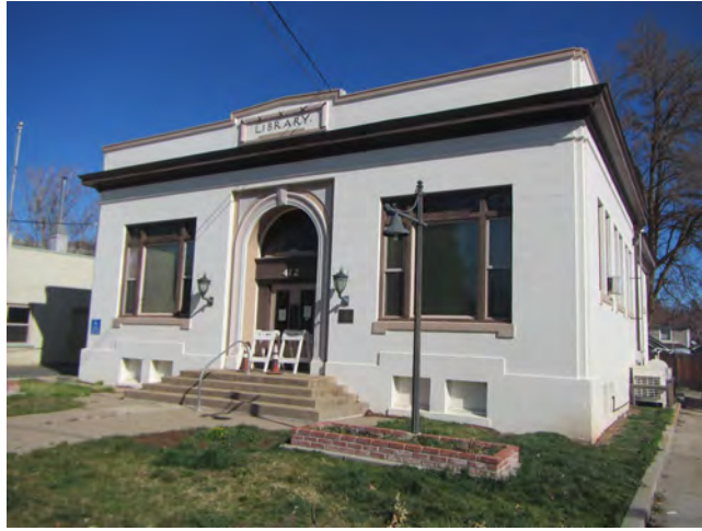
Photo 1 – Yreka Library building (southern exterior), 412 West Miner Street, Yreka, Siskiyou County, California
