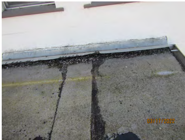
Photo 27 – Asphalt built-up roofing, portico roof, northern office entrance
