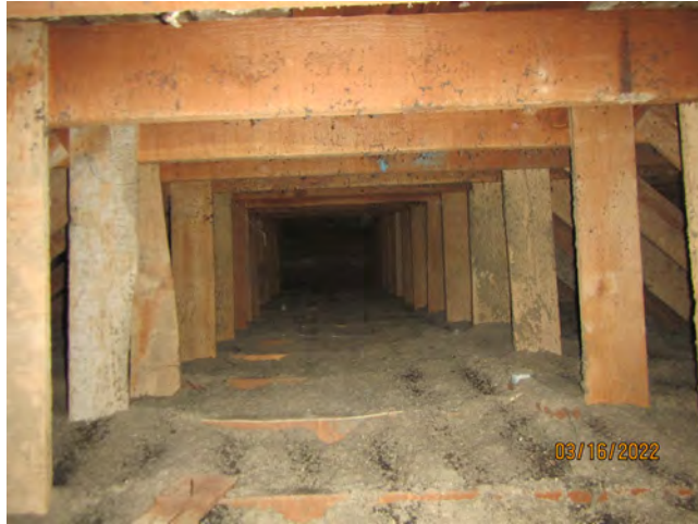
Photo 19 – Gray flock insulation, 1 st floor ceiling cavity, southern offices
