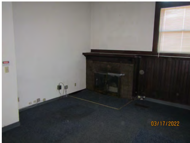
Photo 20 – Typical plaster perimeter wall, southern offices
