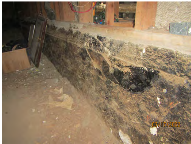
Photo 23 – Black vapor barrier, concrete foundation walls, crawlspace, southern offices
