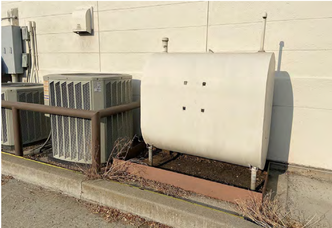
Photo No. 7 Kerosene AST in secondary containment on eastern side of site building
