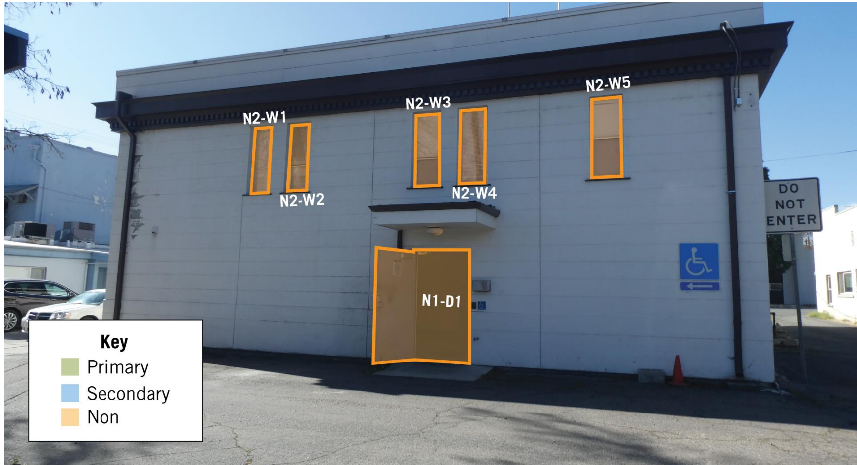
Figure 12: Windows and doors on north elevation. (GPA Consulting, March 2022).
