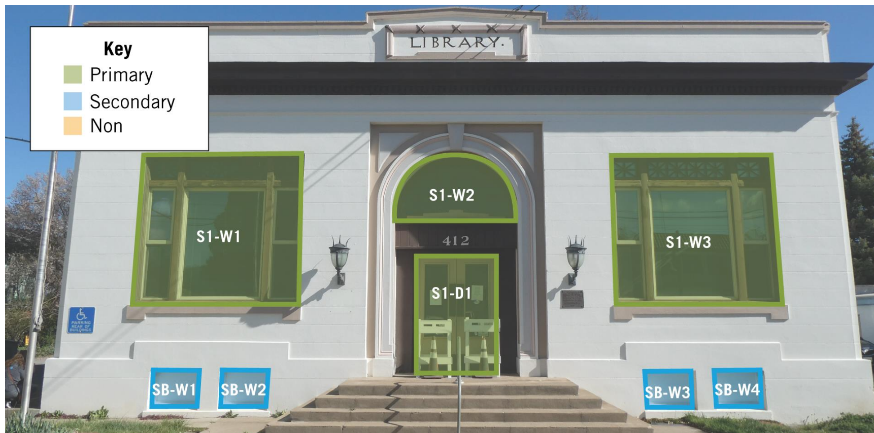
Figure 10: Windows and doors on south elevation. (GPA Consulting, March 2022).
